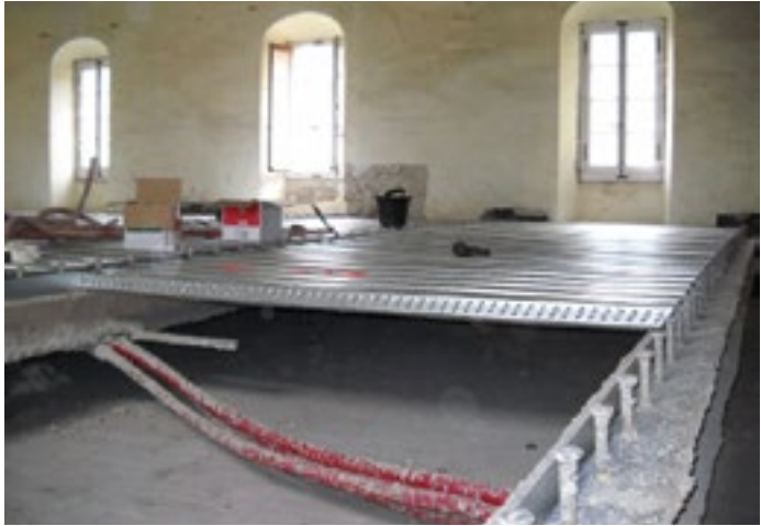
Installation within rehabilitation project - Cofraplus® 60
