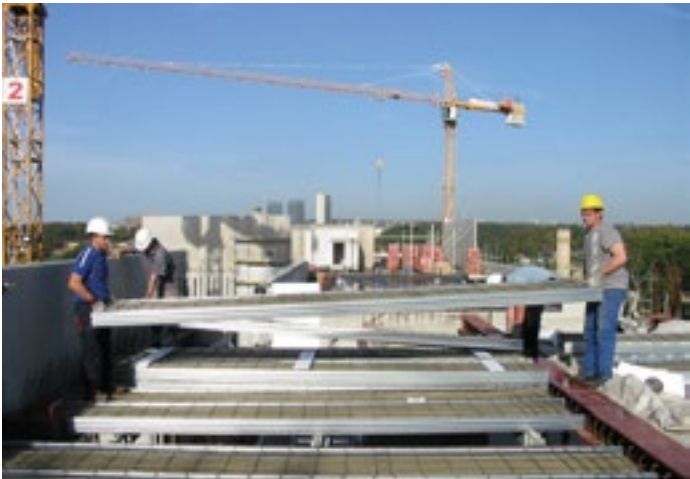
Installation of Cofradal® 200
