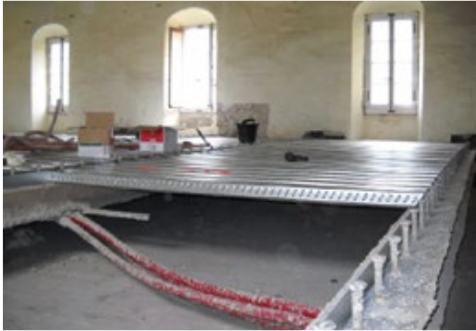
Installation within rehabilitation project - Cofraplus® 60
